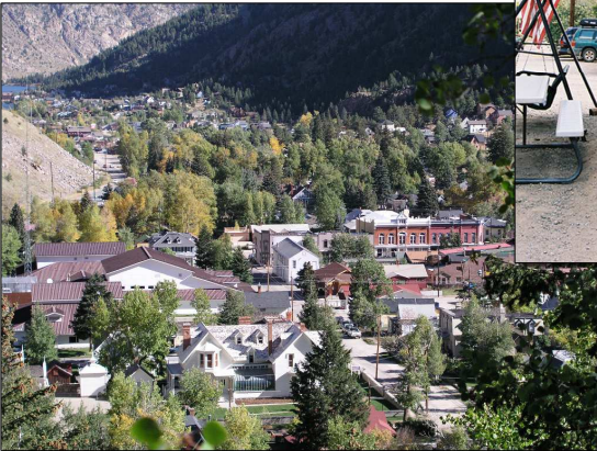
VIEW SOUTHEAST ACROSS GEORGETOWN
